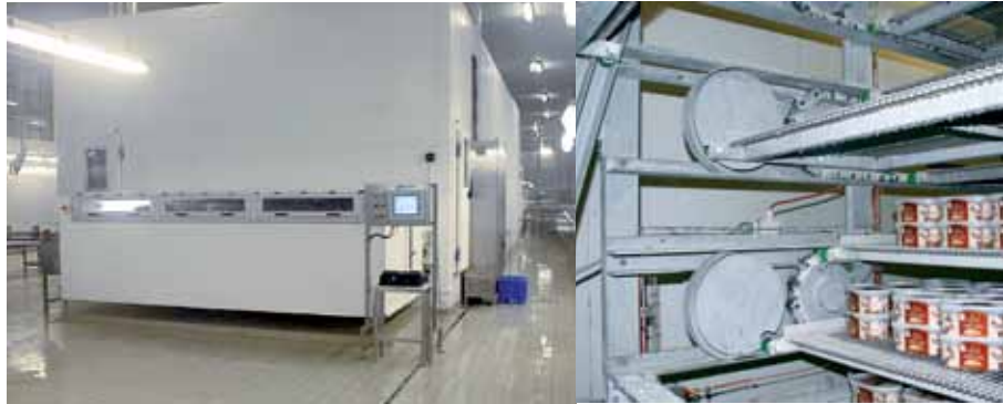
HJ40 Tray Tunnel behind the isolated white walls, and the front shows the stainless steel enclosure with electrical controls easy to operate on a finger-touch screen. The picture to the right gives a peek into one of the turning stations in HJ40.
