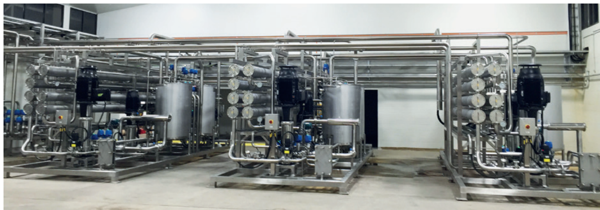
Reverse Osmosis plant from GEA.
