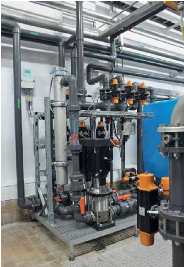
Fully automatic CIP (Cleaning-In-Place) unit in order to perform regular cleaning of the membranes to remove precipitations caused by calcium salts or bio-fouling.
