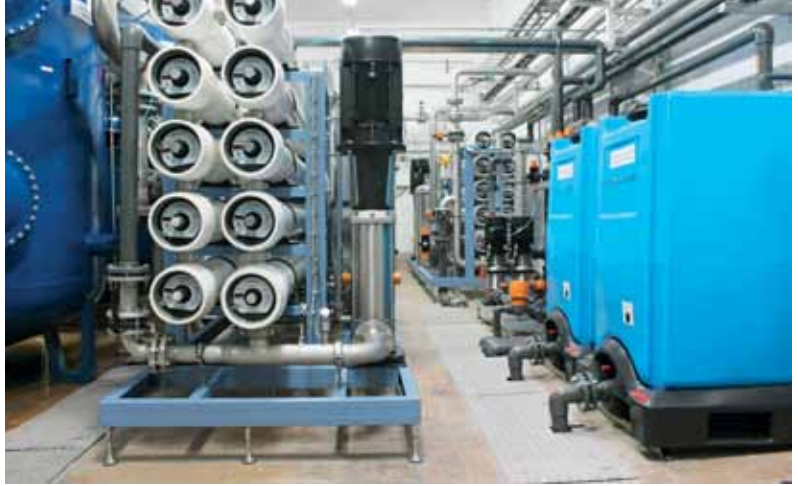
Water treatment plant at PepsiCo / Wimm-Bill-Dann dairy in Kiev, Ukraine. Left: Multimedia filters. Middle: reverse osmosis units. Right: Automatic CIP unit. Projecting and installation done by EUROWATER in Ukraine.
